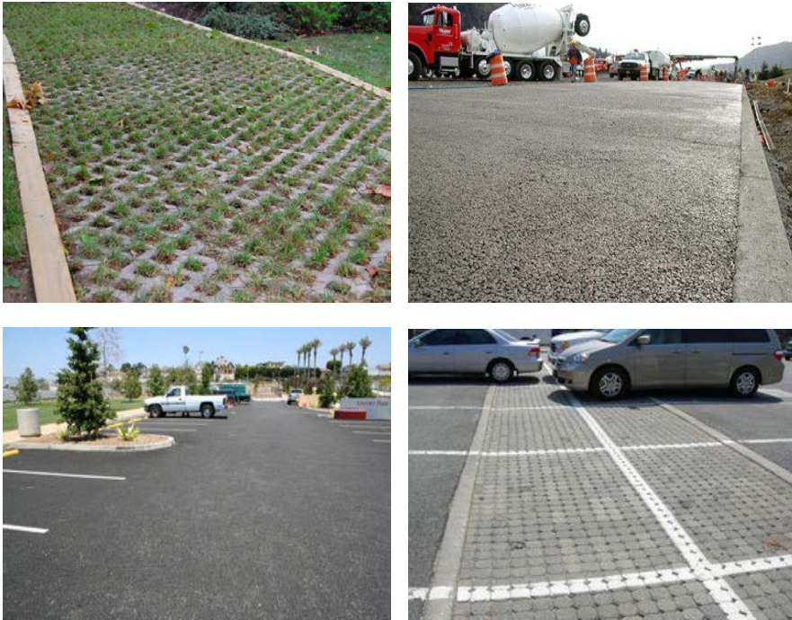
Figure 7.1. Types of Permeable Pavement: (clockwise from upper left): Concrete Grid Pavers (Chesapeake Stormwater Network); Pervious Concrete ( www.perviouspavement.org ), Porous Asphalt (UC Davis) Permeable Interlocking Concrete Pavers (UC Davis)
