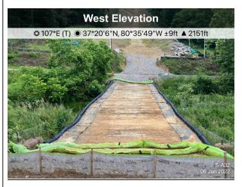
Figure 4: St 10890 ECD's and stabilization in place.
