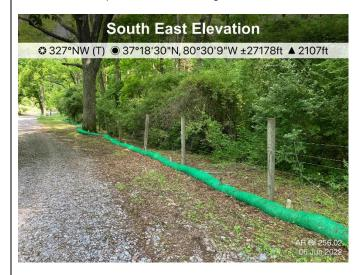
Figure 2: St10877 ECD's and stabilization in place.
