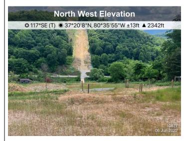
Figure 3: Designated crossing S-A32, ESC's are in place and functioning.
