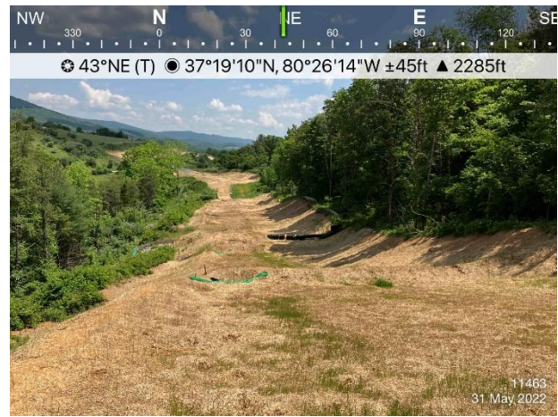
Figure 4: St11463 ECD's and stabilization in place.
