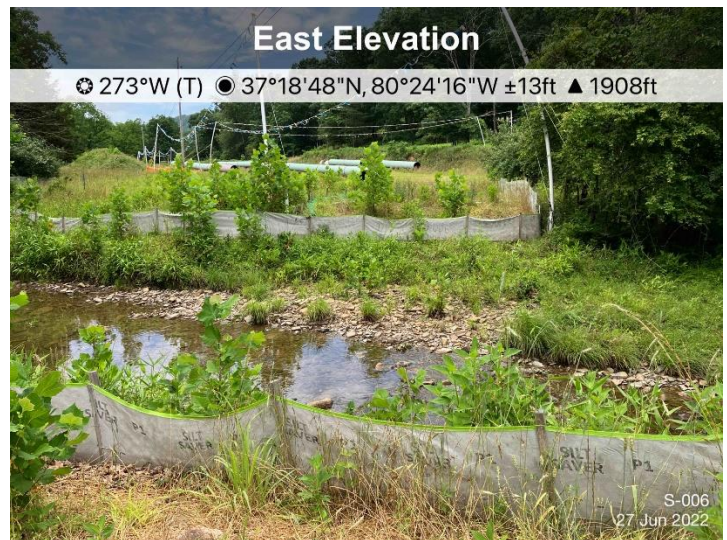
Figure 4: Designated crossing S-006, ESC's are in place and functioning.
