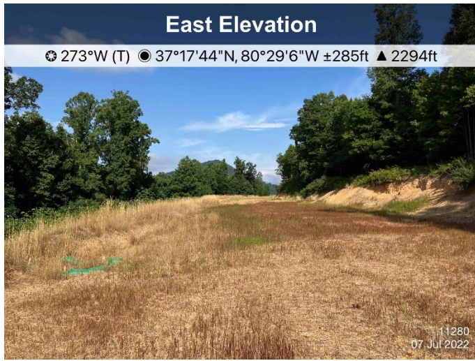
Figure 1: St11280, ECD's and stabilization are in place.
