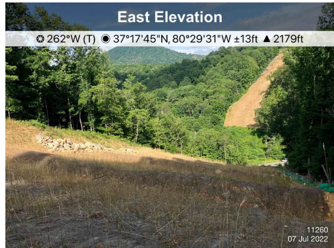
Figure 2: St11260, ECD's and stabilization are in place
