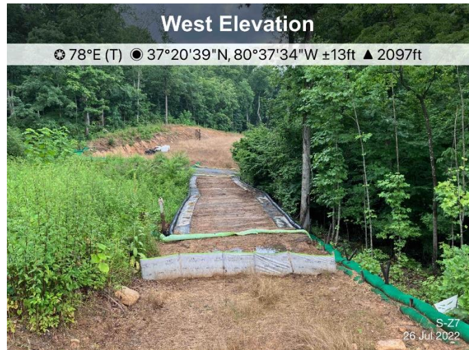
Figure 2: Designated crossing S-Z7, ECD's are in place.
