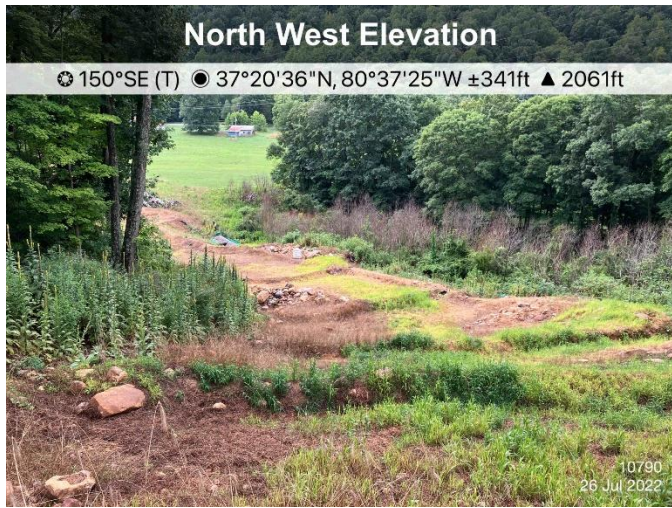
Figure 1: St10790, ECD's and stabilization are in place.
