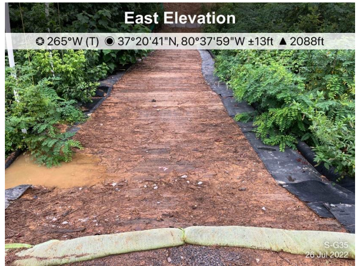
Figure 4: Designated crossing S-G35, ECD's are in place.
