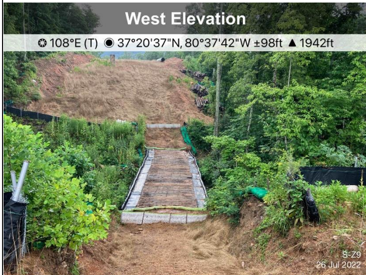
Figure 3: Designated crossing S-Z9, ECD's are in place.
