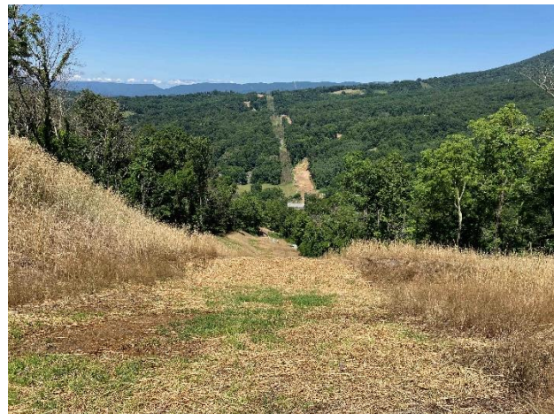
Figure 2: St10819, ECD's and stabilization are in place
