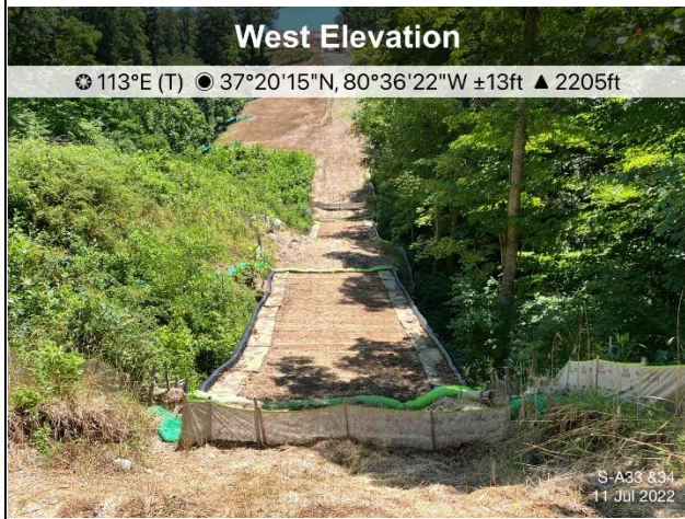
Figure 3: Designated crossing S-A33&34, ECD's are in place.
