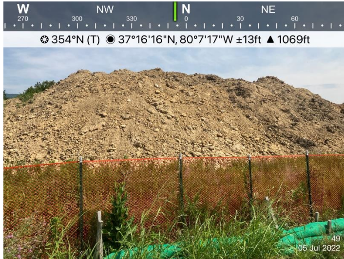
Figure 5: Laydown Yard 049 – Looking N towards offsite un-stabilized stockpiles. No controls around the stockpiles.
