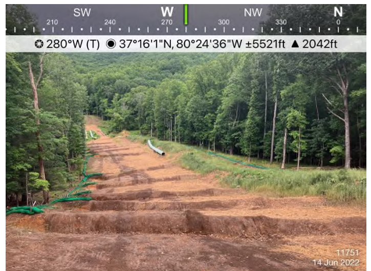
Figure 4: STA 11751+00 – Controls in place and functioning properly. Area stabilized with straw.
