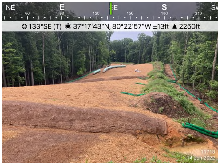
Figure 3: STA 11718+00 – Controls in place and functioning properly. Area stabilized with straw.
