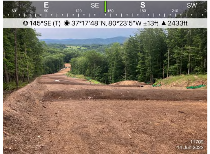
Figure 4: STA 11751+00 – Controls in place and functioning properly. Area stabilized with straw.
