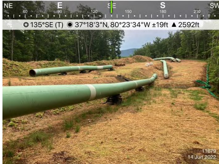
Figure 3: STA 11718+00 – Controls in place and functioning properly. Area stabilized with straw.
