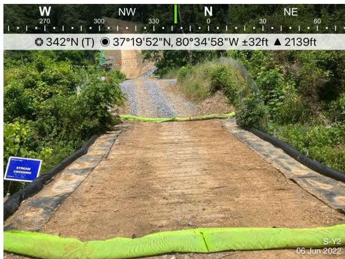
Figure 3: Stream S-Y2 – Controls in place and functioning properly along stream crossing.
