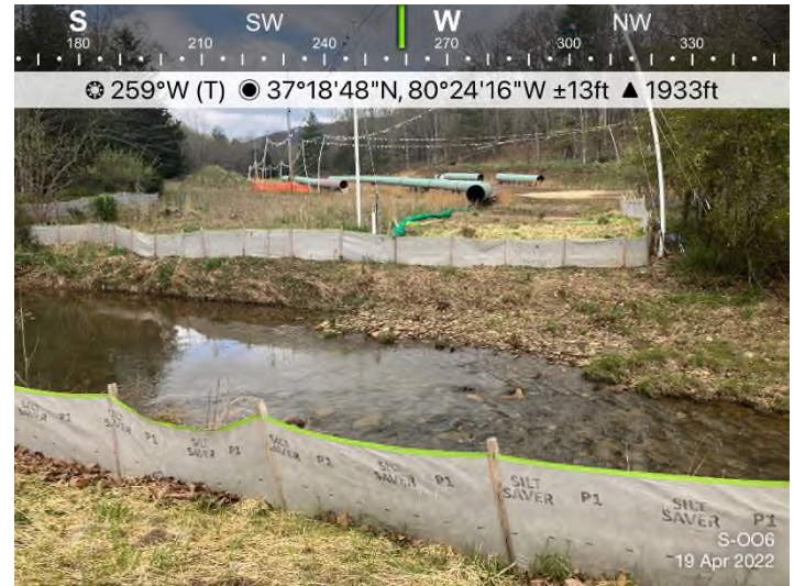
Figure 4: Stream S-RR14 – Controls in place and functioning properly along stream crossing.
