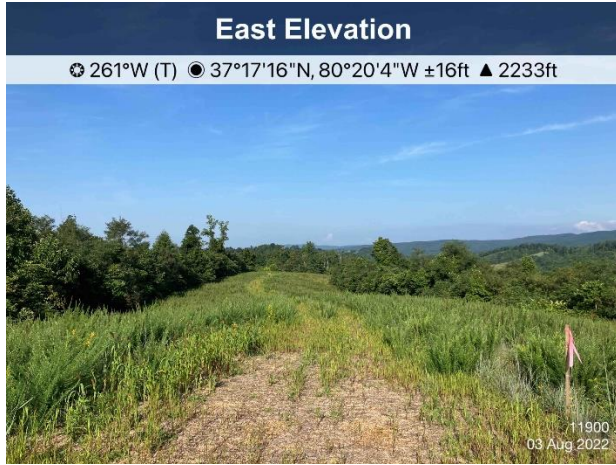
Figure 1: St11900 ECD's and stabilization are in place.
