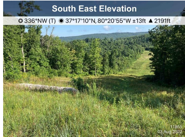
Figure 2: St11855, ECD's and stabilization are in place.
