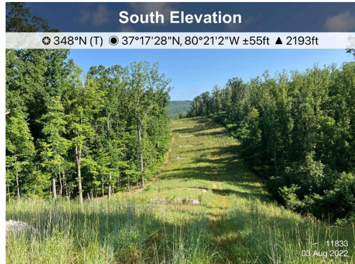
Figure 4: St11833, ECD's and stabilization are in place.
