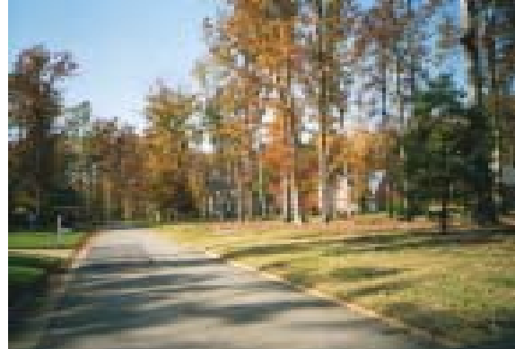
Figure 5.6: Instead of a traditional cul-de-sac, West Whittaker Close is a loop-de-lane -- a road with a 16-foot one-way travel lane and a 90-foot central landscaped area.
