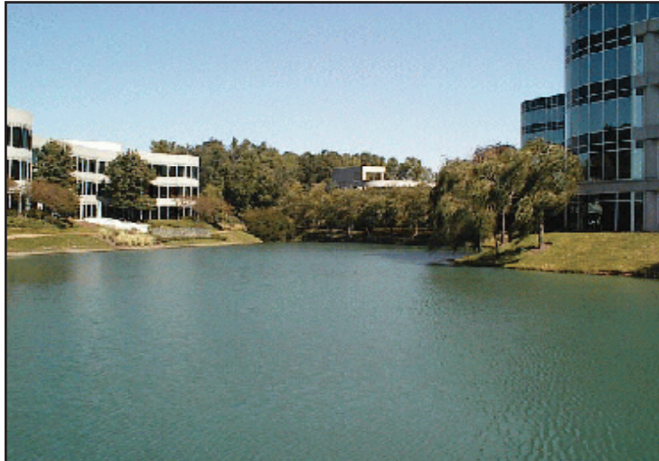
Figure 7.1: Regional stormwater management facility with Arboretum I on the left, Arboretum III on the right, and the Arboretum III parking structure in the background.
