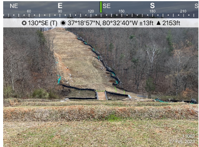
Figure 4: St 11062 ECD's are in place.
