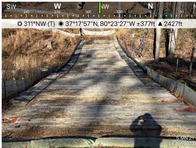
Figure 3: Designated crossing S-MN21, ECD's are in place.
