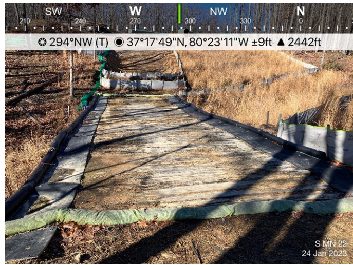
Figure 4: Designated crossing S-MN22, ECD's are in place.
