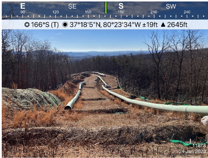
Figure 1: St11678, area is stabilized and ECD's are in place.
