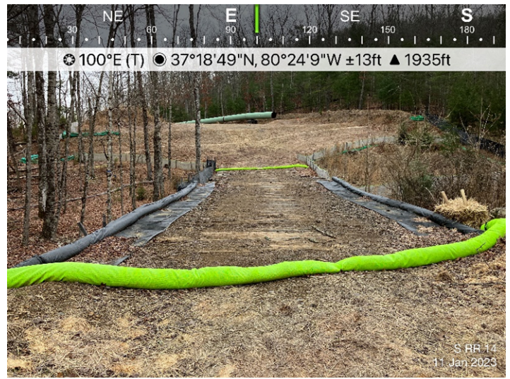
Figure 4: Designated crossing S-RR14, ECD's are in place.
