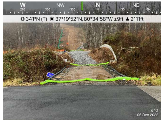
Figure 4: Designated crossing S-Y2, ECD's are in place.
