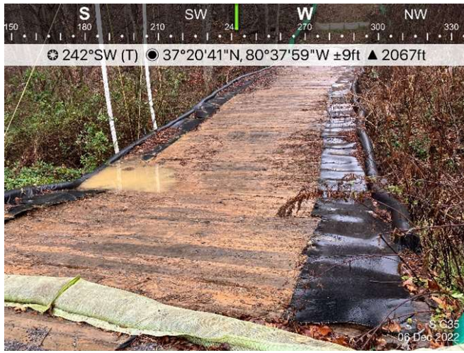
Figure 1: St G35, area is stabilized and ECD's are in place.
