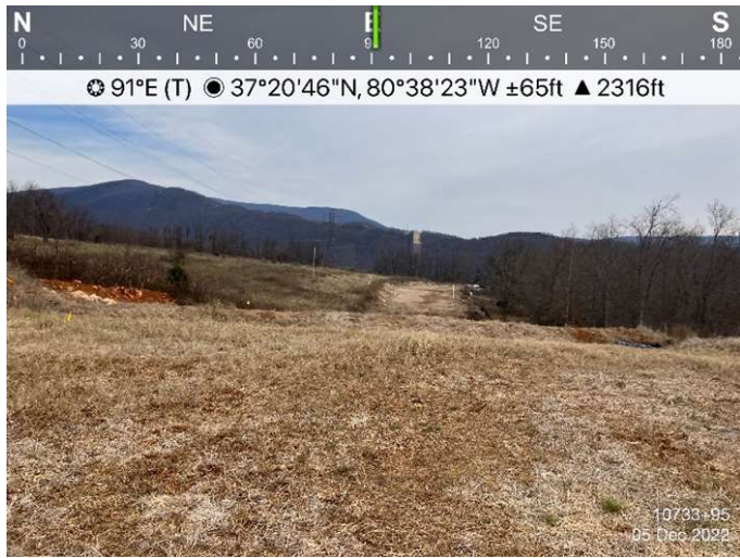
Figure 1: St 10733+95, area is stabilized and ECD's are in place.
