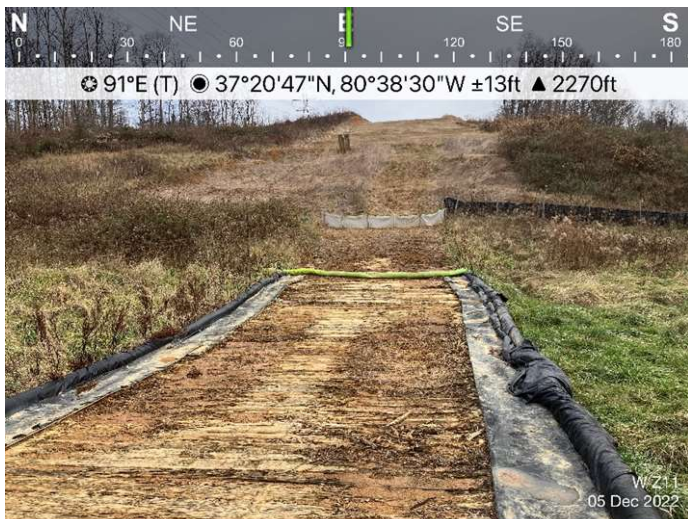
Figure 3: Designated crossing W-Z11, ECD's are in place.
