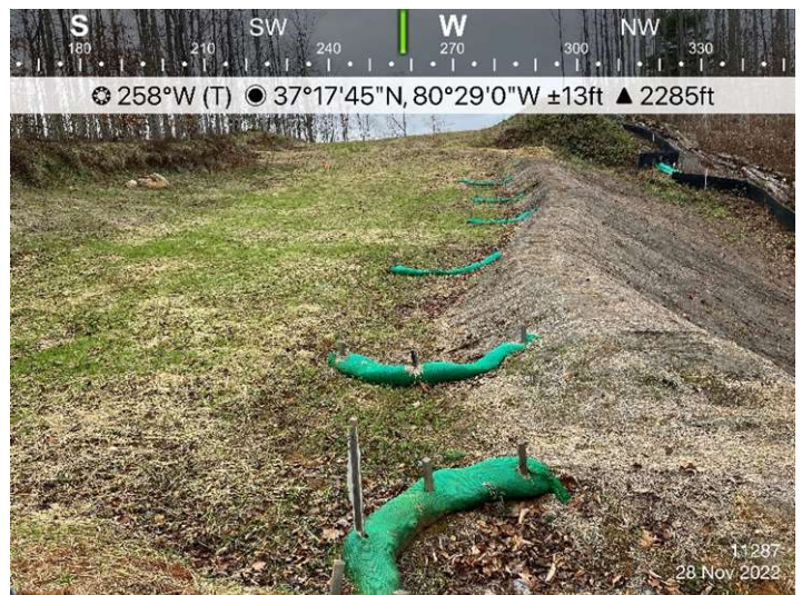
Figure 4: St11287, area is stabilized and ECD's are in place.
