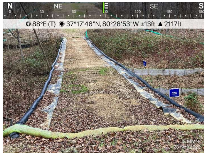
Figure 2: Designated crossing S-MM18, ECD's are in place.
