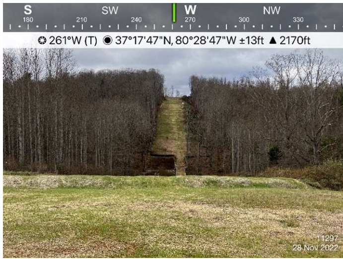
Figure 1: St11297, area is stabilized and ECD's are in place.
