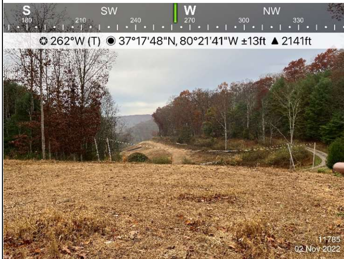
Figure 3: St 11785, area is stabilized and ECD's are in place.
