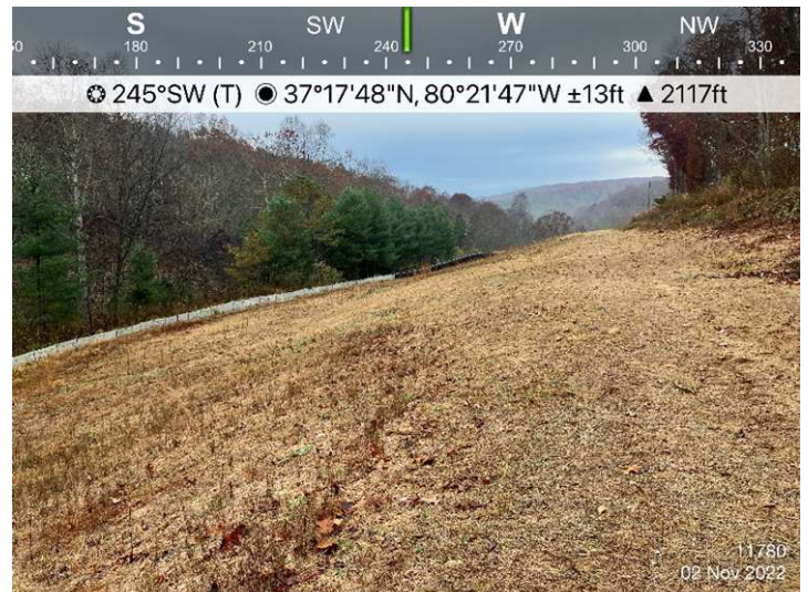
Figure 4: St 11780, area is stabilized and ECD's are in place.
