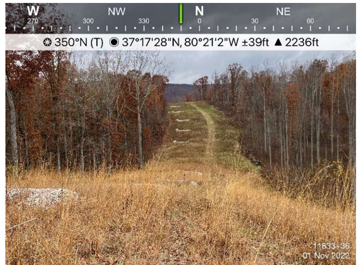
Figure 4: St 11833+36, area is stabilized and ECD's are in place.
