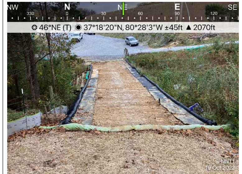
Figure 2: Designated crossing S-NN11, ECD's are in place.
