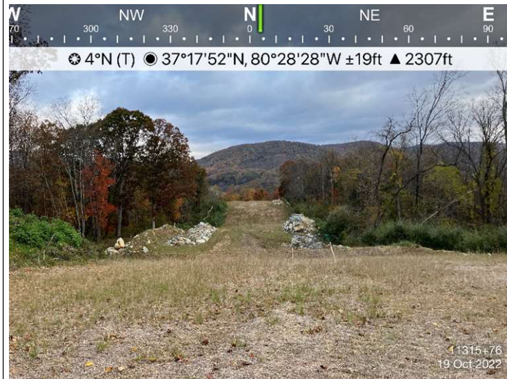
Figure 1: St11315+76, area is stabilized and ECD's are in place.
