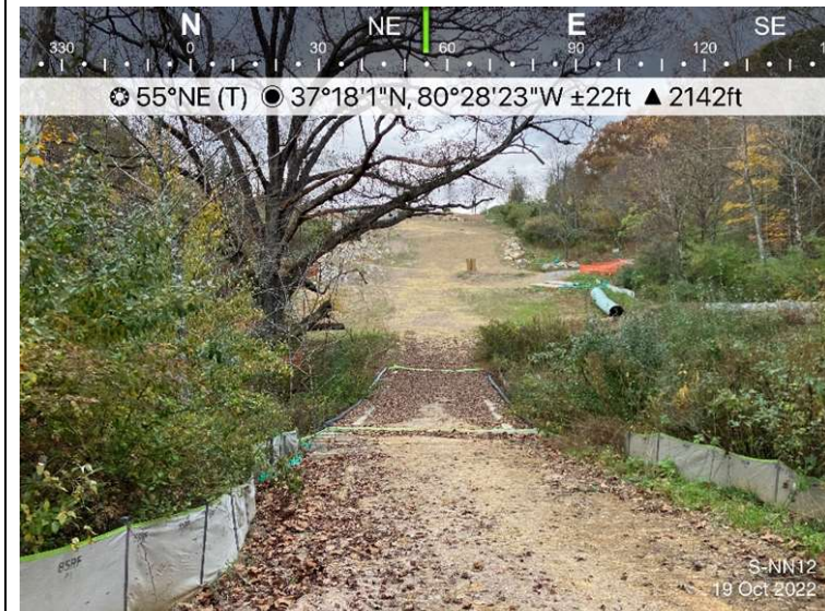
Figure 3: Designated crossing S-NN12, ECD's are in place.
