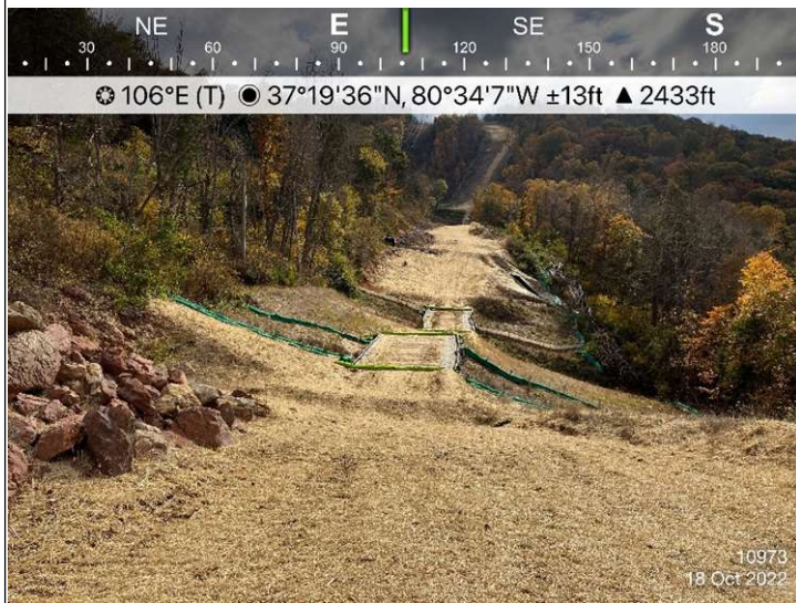
Figure 1: St10973, area is stabilized and ECD's are in place.
