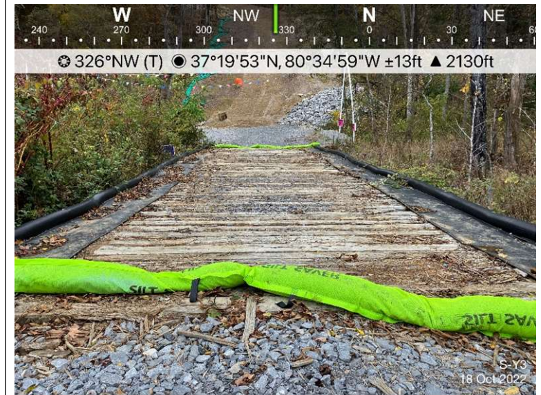
Figure 2: Designated crossing S-Y3 ECD's are in place.
