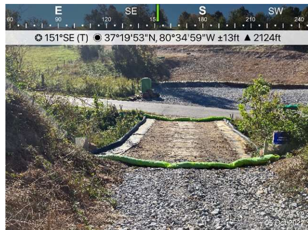
Figure 3: Designated crossing S-Y2, ECD's are in place.
