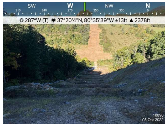
Figure 4: St10890, area is stabilized and ECD's are in place.
