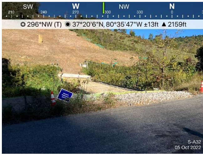
Figure 1: Designated crossing S-A32, ECD's are in place.
