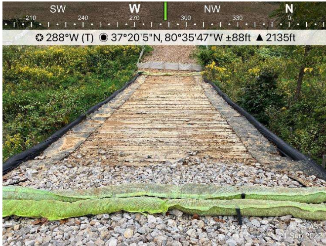
Figure 1: Designated crossing S-A32, ECD's are in place.
