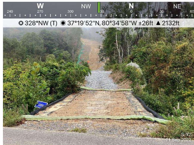
Figure 4: Designated crossing S-Y2, ECD's are in place.
