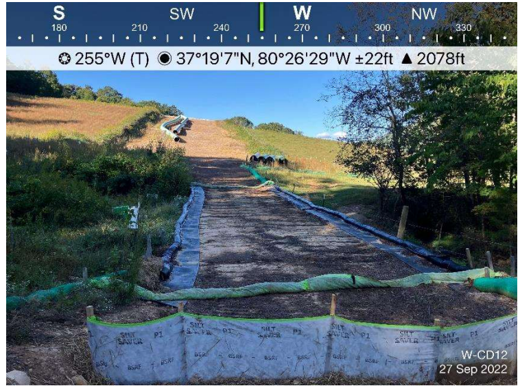
Figure 2: Designated crossing W-CD12, ECD's are in place.
