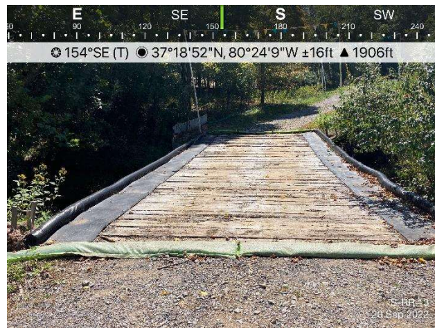
Figure 4: Designated crossing S-RR13, ECD's are in place.
