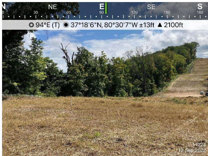
Figure 3: St11224, ECD's and stabilization are in place.
