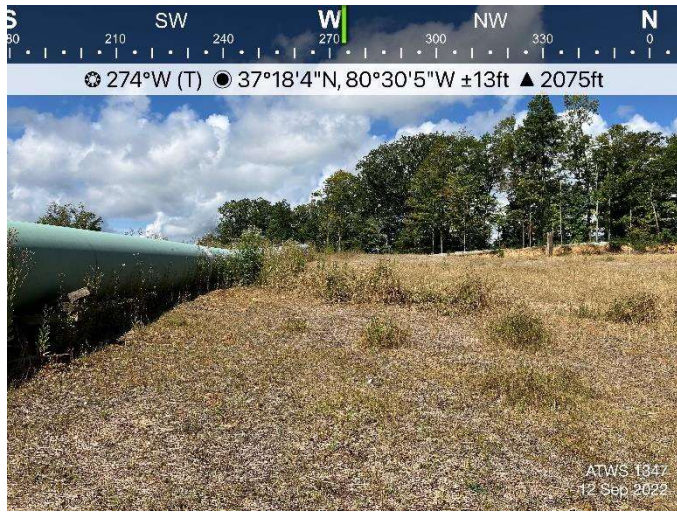
Figure 1: ATWS 1347, ECD's and stabilization are in place.
