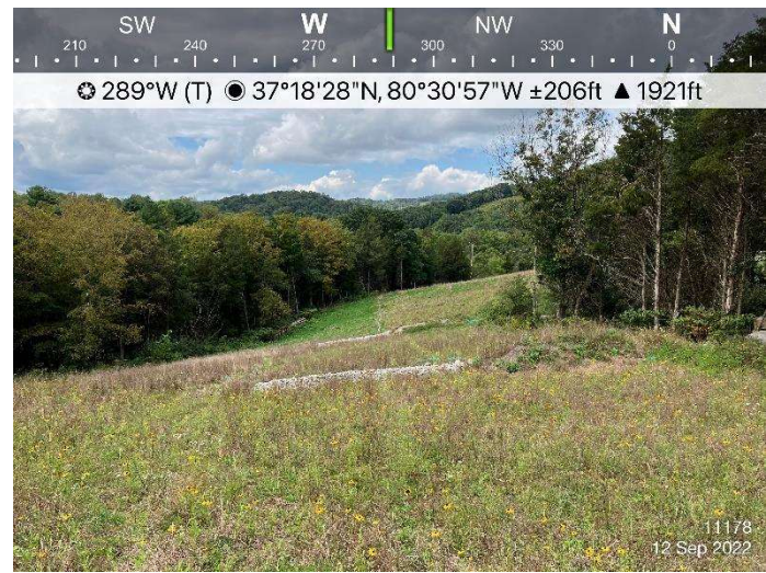
Figure 4: St11178, ECD's and stabilization are in place.
