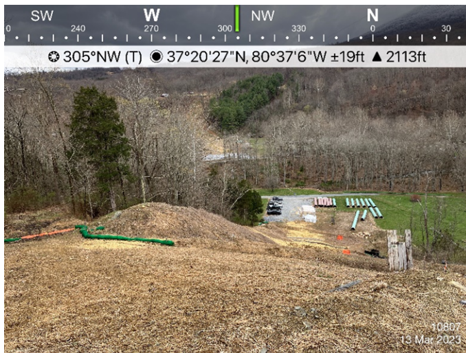
Figure 3: St10807 ECD's are in place.
