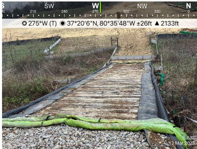
Figure 1: Designated crossing S-A32, ECD's are in place.
