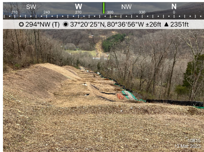
Figure 4: St10815 ECD's are in place.
