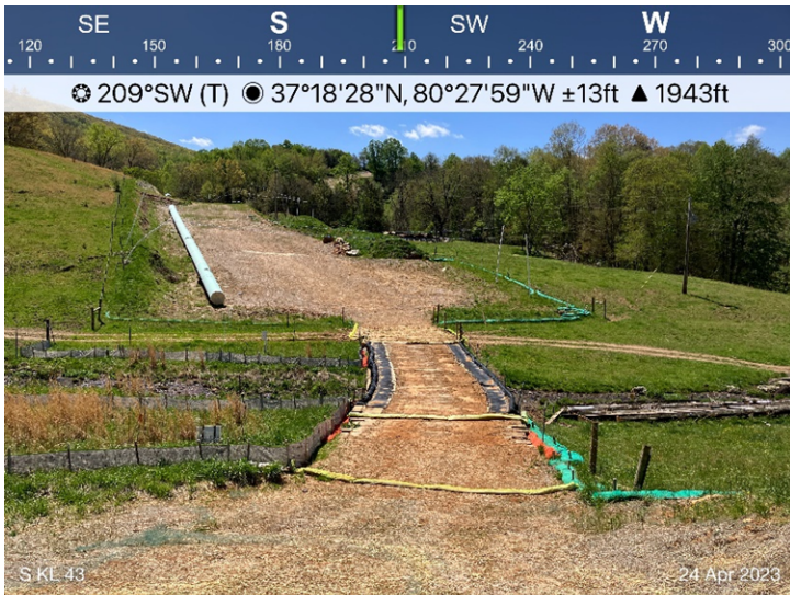
Figure 3: Designated crossing S-KL43, ECD's are in place.
