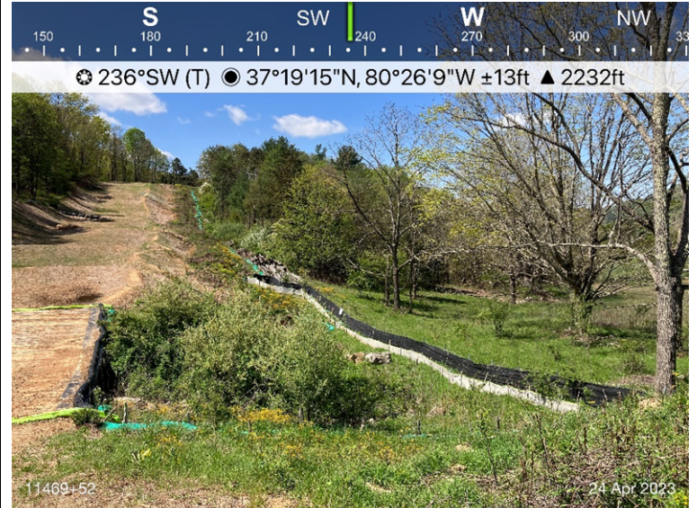
Figure 2: Sta 11469+52, ECD's in place.
