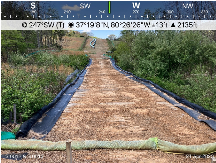
Figure 1: Designated crossing S-0012 & S-0013, ECD's are in place.
