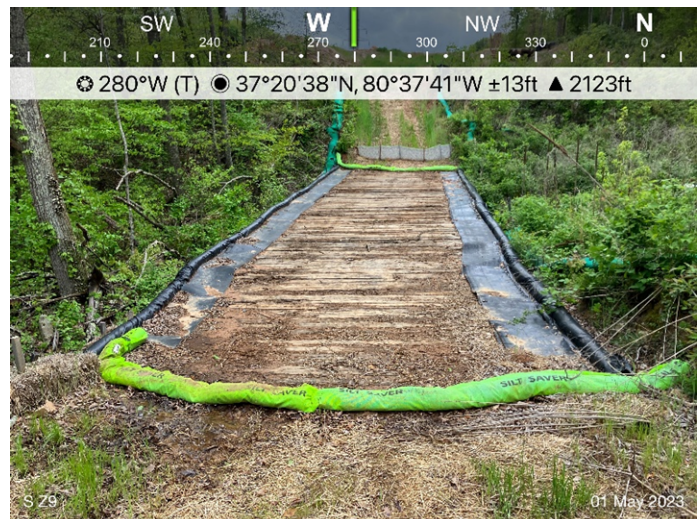
Figure 4: Designated crossing S-Z9, ECD's are in place.
