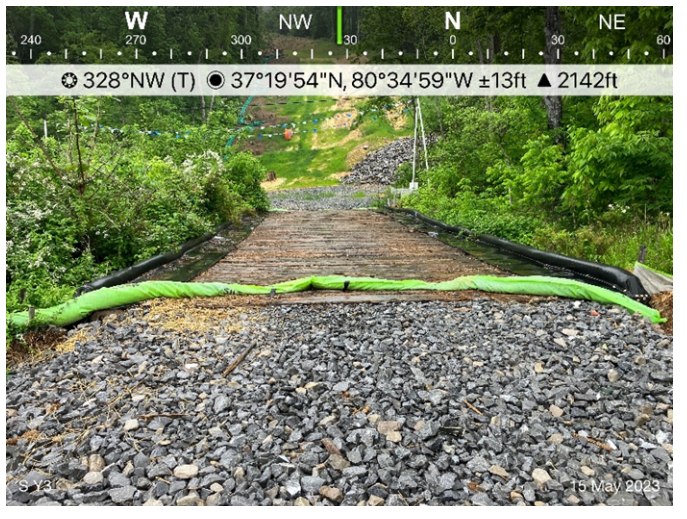
Figure 4: Designated crossing S-Y3, ESC measures in place.
