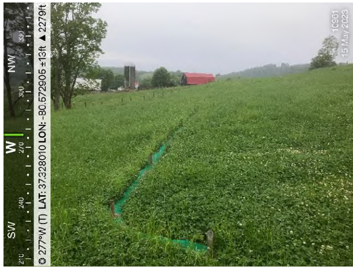
Figure 3: STA 10950+00 – Permanent vegetative cover established. Ground cover is uniform, mature enough to survive and will inhibit erosion.
