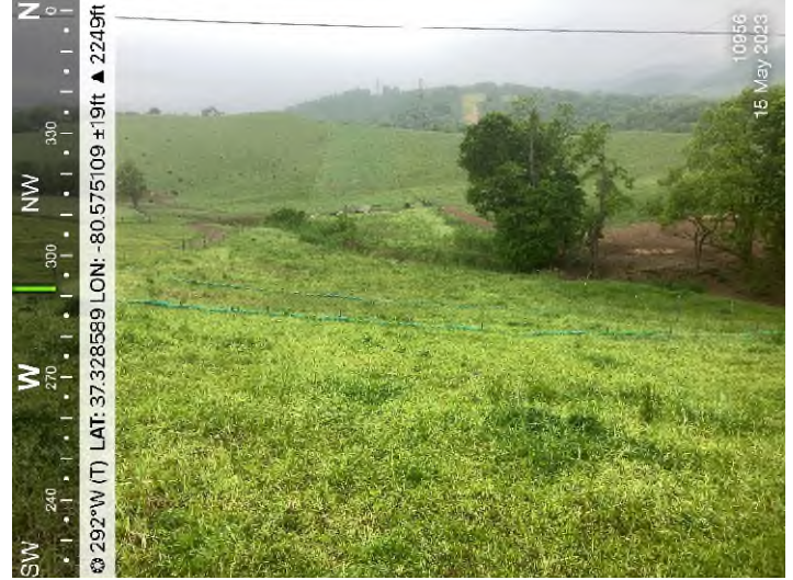
Figure 2: STA 10956+00 – Permanent vegetative cover established. Ground cover is uniform, mature enough to survive and will inhibit erosion.
