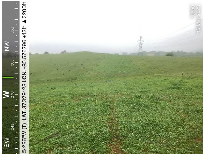
Figure 3: STA 10950+00 – Permanent vegetative cover established. Ground cover is uniform, mature enough to survive and will inhibit erosion.
