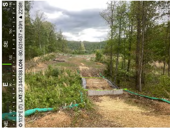
Figure 3: STA 10787+00 – Controls in place and functioning properly.
