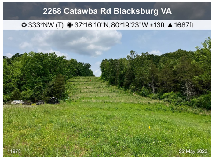
Figure 4: Sta 11978 ECD's and stabilization are in place.
