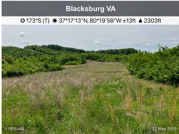
Figure 1: Sta 11905+68 ECD's and stabilization are in place.
