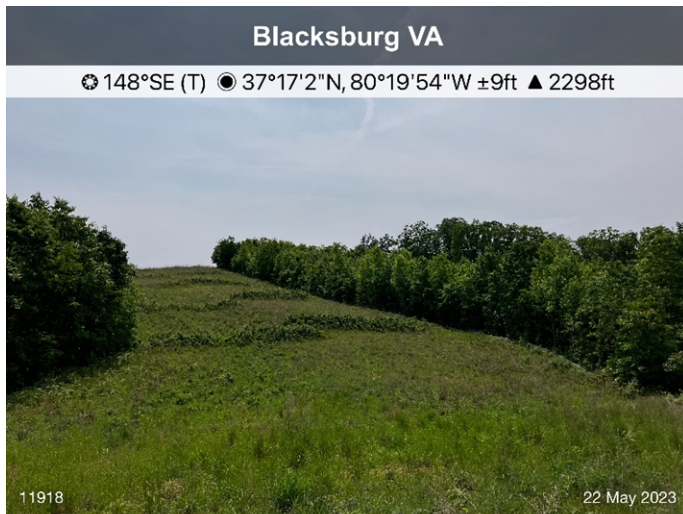
Figure 3: Sta 11918 ECD's and stabilization are in place.
