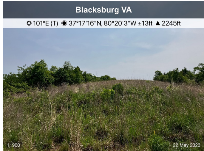
Figure 2: Sta 11900 ECD's and stabilization are in place.
