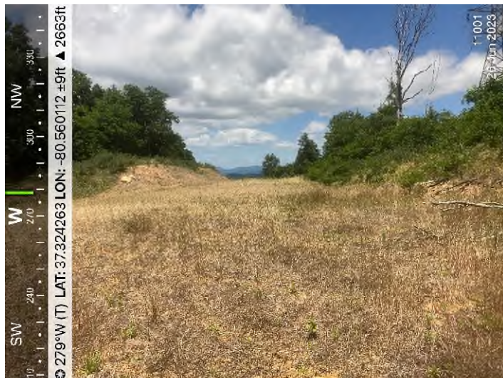
Figure 3: STA 11001+00 – Controls in place and functioning properly.
