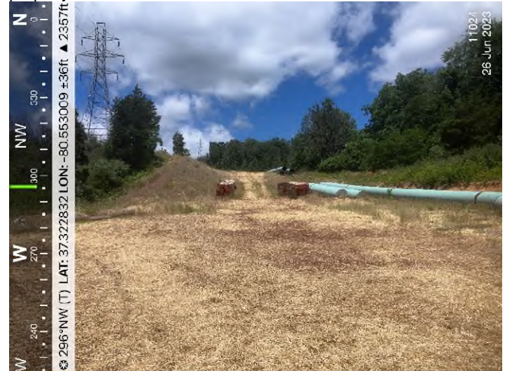
Figure 2: STA 11024+00 – Controls in place and functioning properly. Area stabilized with straw.
