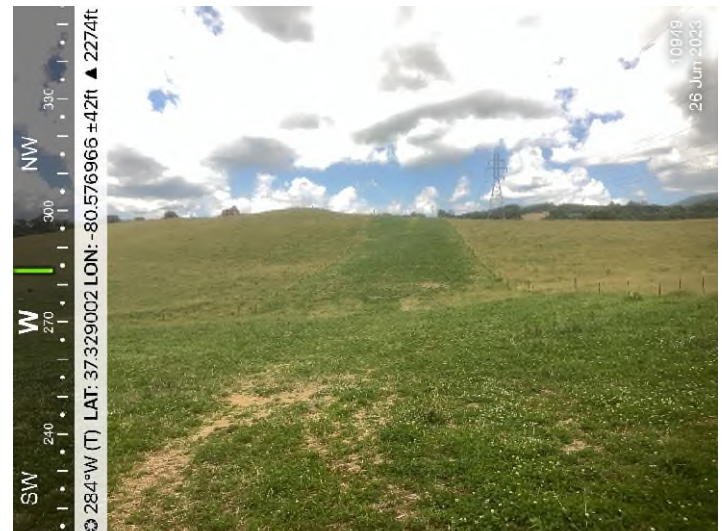
Figure 4: STA 10949+00 – Controls in place and functioning properly. Area at final grade.
