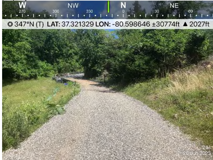
Figure 1: MVP-GI-244 – Controls in place and functioning properly.
