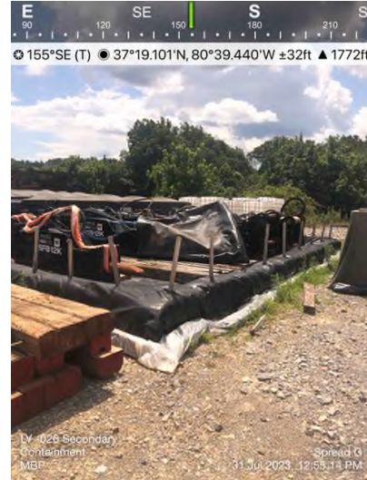
Figure 2: Laydown Yard 026 – Controls in place and functioning properly.
