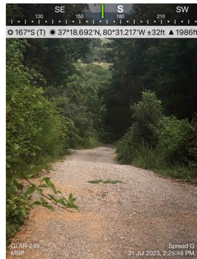
Figure 4: MVP-GI-249 – Controls in place and functioning properly.
