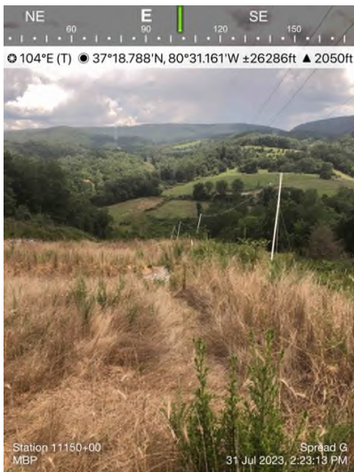
Figure 3: STA 11150+00 – Controls in place and functioning properly.
