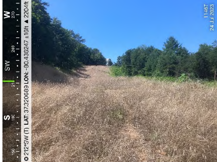
Figure 1: STA 11467+00 – Controls in place and functioning properly.
