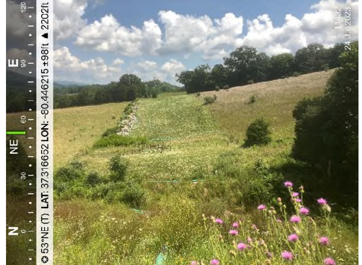
Figure 2: STA 11432+00 – Controls in place and functioning properly.
