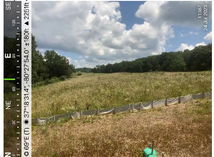
Figure 4: STA 11367+00 – Controls in place and functioning properly.
