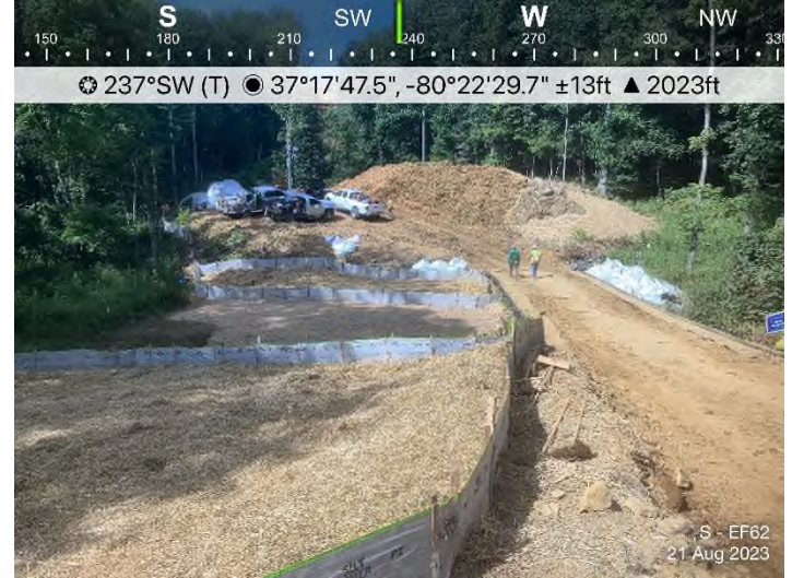
Figure 2: Stream S-EF62 – Controls in place and functioning properly.
