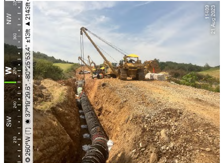
Figure 4: STA 11489+00 – Controls in place and functioning properly.
