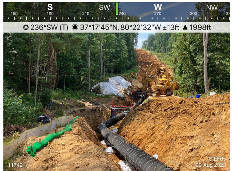
Figure 4: Designated crossings S-EF65, ECD's are in place.
