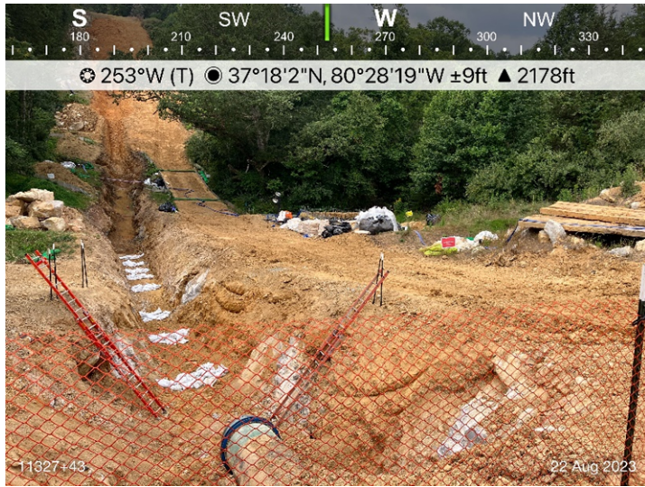
Figure 1: Designated crossing S-NN12, ECD's are in place.
