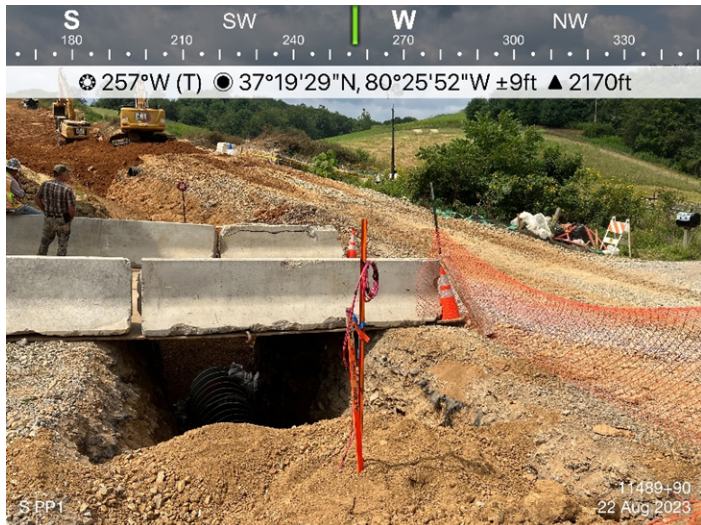
Figure 3: Designated Crossing S-PP1, ECD's are in place for active construction.
