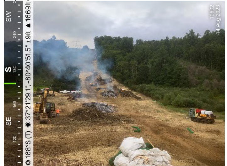
Figure 2: STA 10602+00 – Controls in place and functioning properly.
