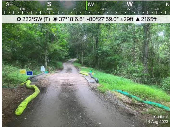
Figure 1: S-NN13 – Controls in place and functioning properly along MVP-GI-256.02.
