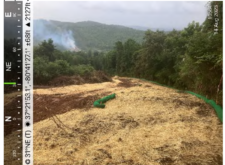
Figure 4: STA 10564+00 – Controls in place and functioning properly.
