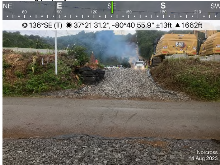
Figure 3: Norcross Road Crossing – Controls in place and functioning properly.
