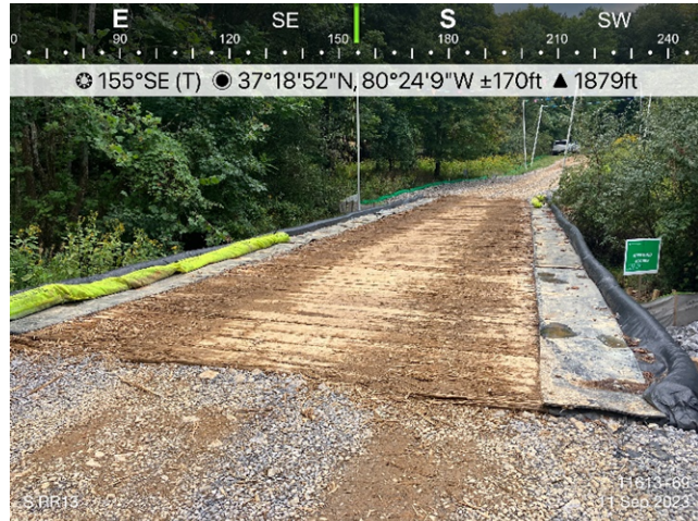
Figure 1: Designated stream S-RR13, ECD's were in place for active construction.
