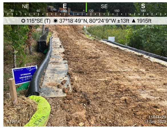
Figure 4: Designated crossing S-RR14, ECD's were in place for active construction.
