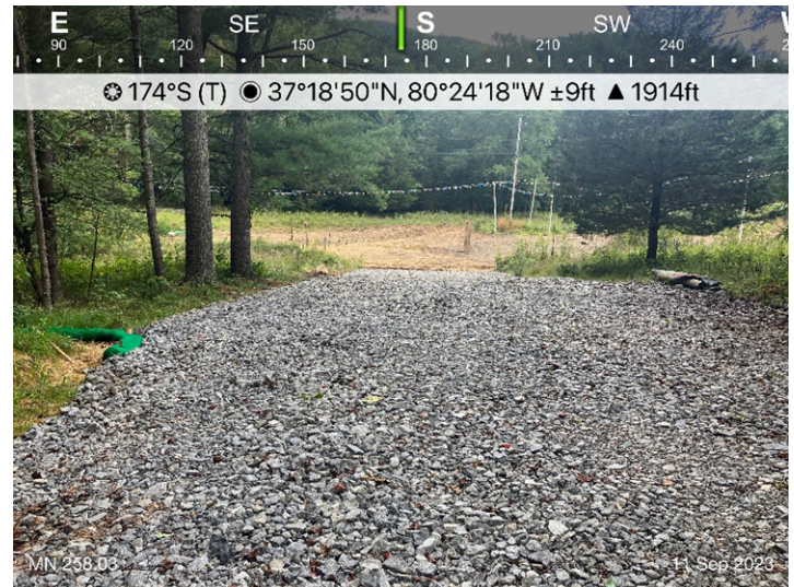
Figure 8: AR MN 258.03, ECD's were in place.
