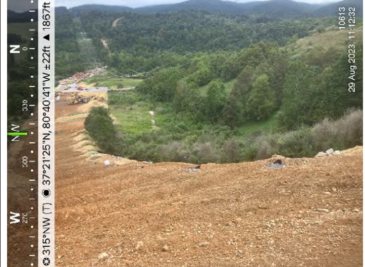
Figure 2: STA 10613+00 – Controls in place and functioning properly.
