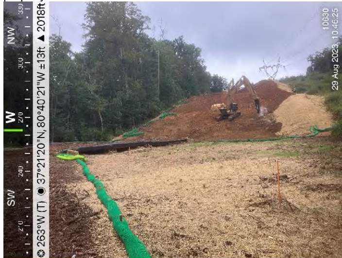
Figure 3: STA 10630+00 – Controls in place and functioning properly.
