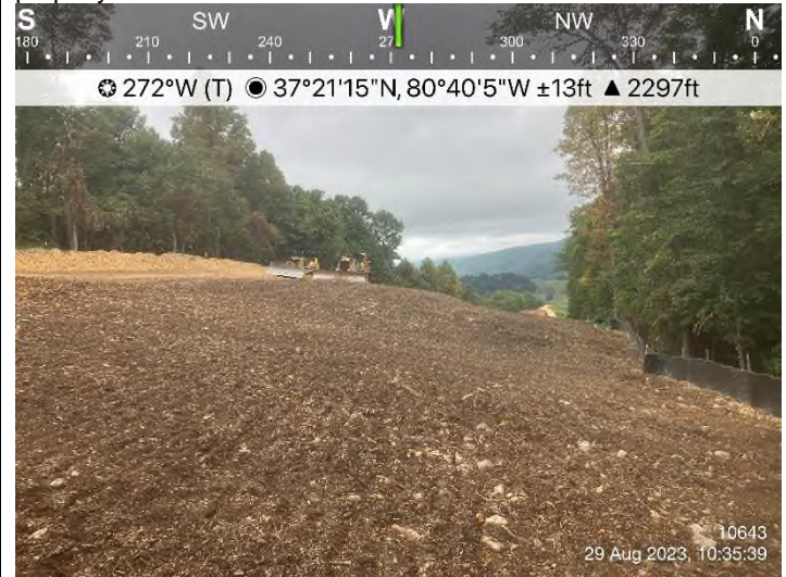
Figure 4: STA 10643+00 – Controls in place and functioning properly.
