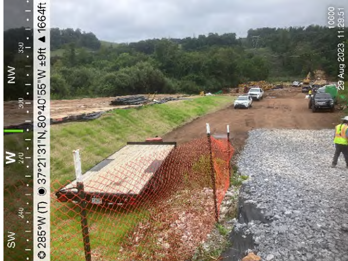
Figure 1: STA 10600+00 – Controls in place and functioning properly.
