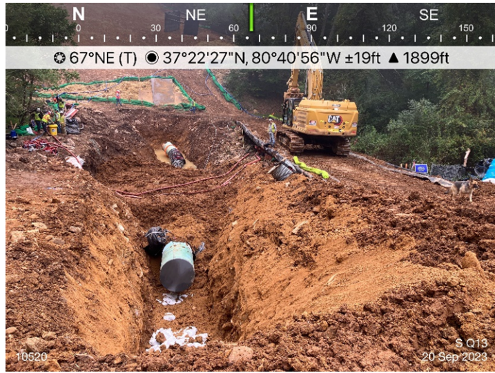
Figure 1: Designated crossing S-Q13, ECD's are in place.
