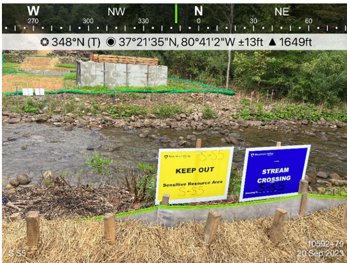
Figure 3: Designated crossing S-S5, ECD's are in place.
