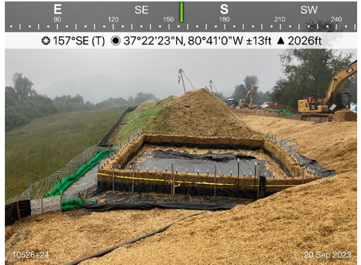
Figure 2: Sta 10526+24, dewatering structure in place.
