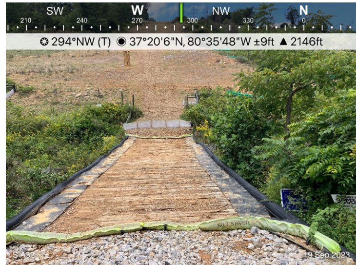
Figure 4: Designated crossing S-A32, ECD's are in place.
