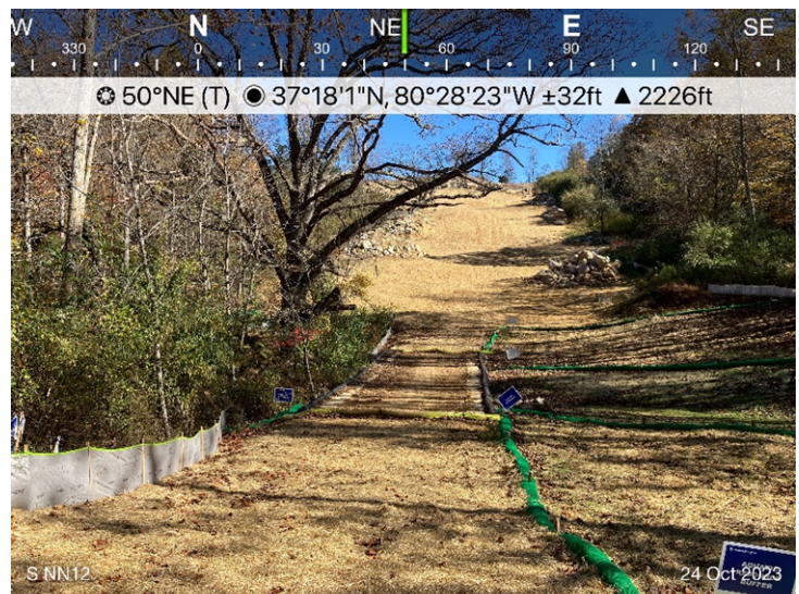
Figure 4: Designated crossing S-NN12, ECD's are in place.
