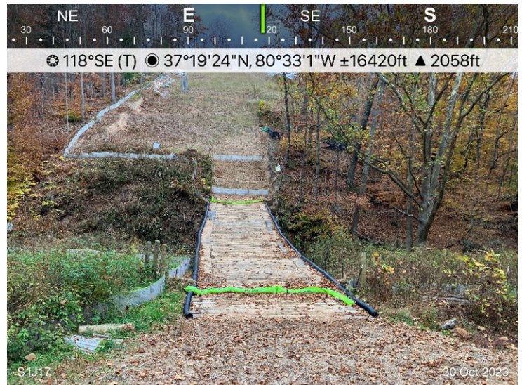
Figure 4: Designated crossing S-IJ17, ECD's are in place.
