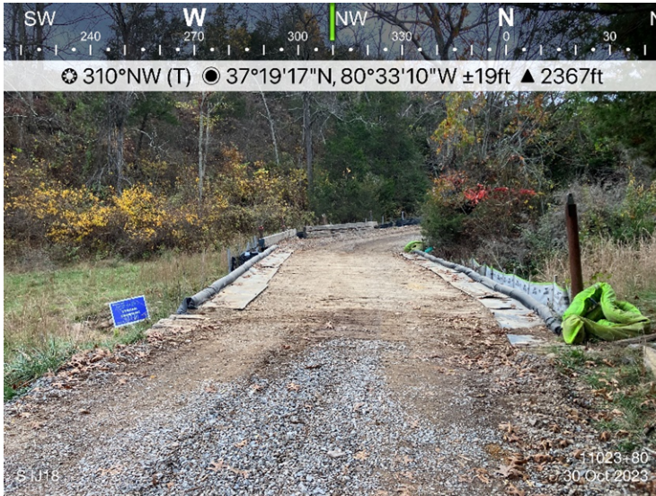
Figure 3: Designated crossing S-IJ19, ECD's are in place for active construction.
