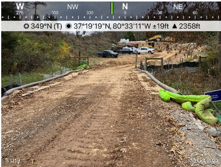
Figure 3: Designated crossing S-IJ19, ECD's are in place for active construction.
