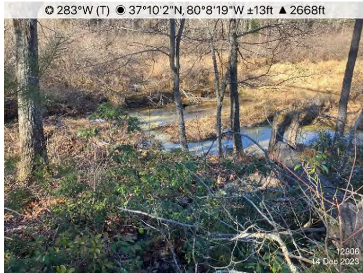
Figure 5: STA 12806+00 – Treated turbid water entering Bottom Creek downstream of the dewatering operation.
