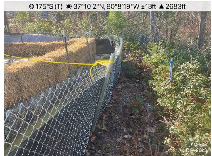
Figure 4: STA 12806+00 – Dewatering structure installed and functioning properly.
