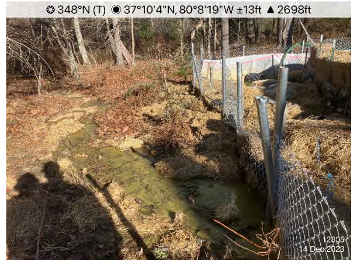
Figure 4: STA 12806+00 – Dewatering structure installed and functioning properly.
