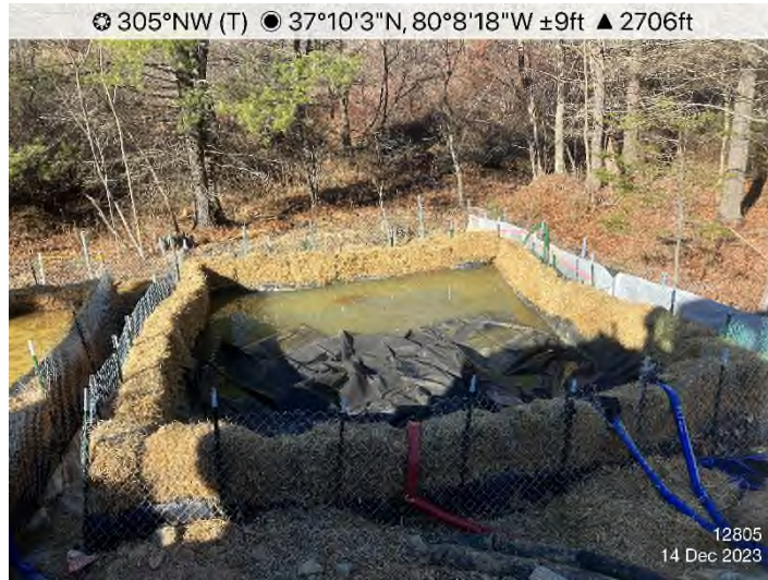
Figure 3: STA 12805+00 – Treated water discharged outside LOD from dewatering structure at STA 12805+00.
