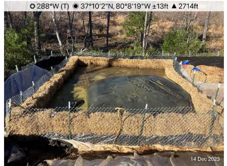
Figure 6: STA 12806+00 – Dewatering structure installed and functioning properly.
