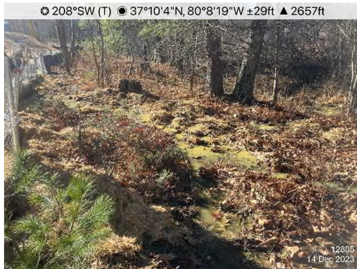
Figure 3: STA 12805+00 – Treated water discharged outside LOD from dewatering structure at STA 12805+00.
