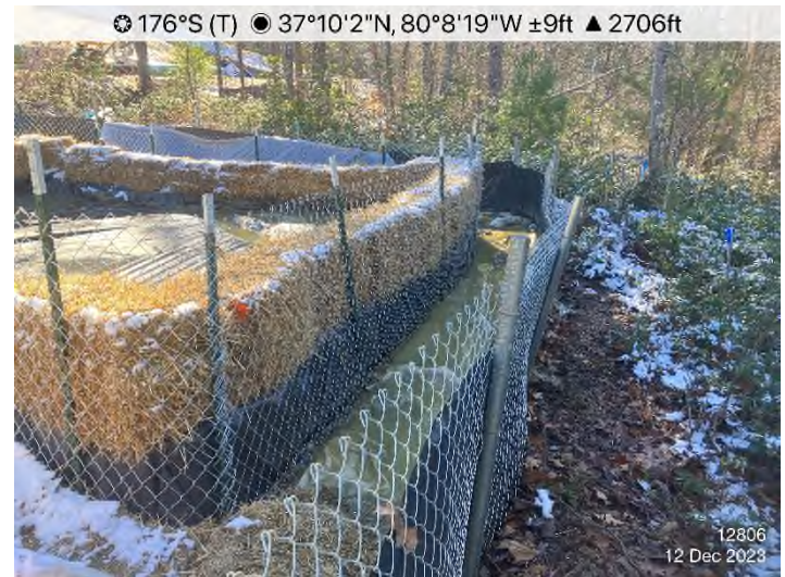
Figure 4: STA 12806+00 – Dewatering structure installed and functioning properly.
