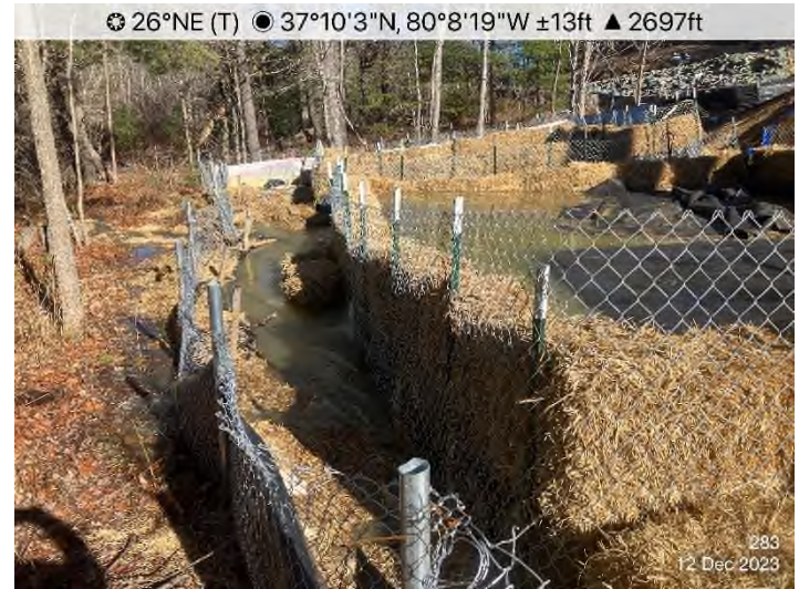
Figure 4: STA 12806+00 – Dewatering structure installed and functioning properly.
