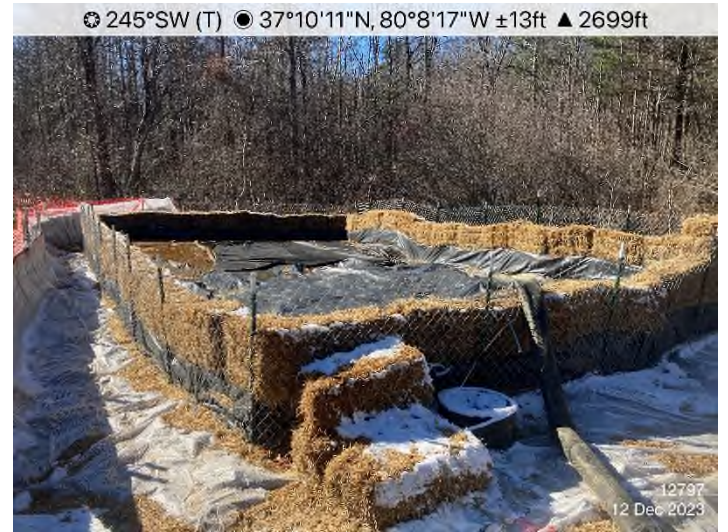
Figure 6: STA 12797+00 – Dewatering structure installed and functioning properly.
