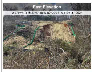
Figure 4: Sta 10525+00, ECD's are in place.
